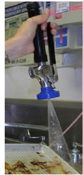
Figure 5: Efficient Spray Valve
