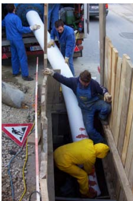
Pipeline renovation using curing-in-place technology. Photo: Roland Rohrhofer.
