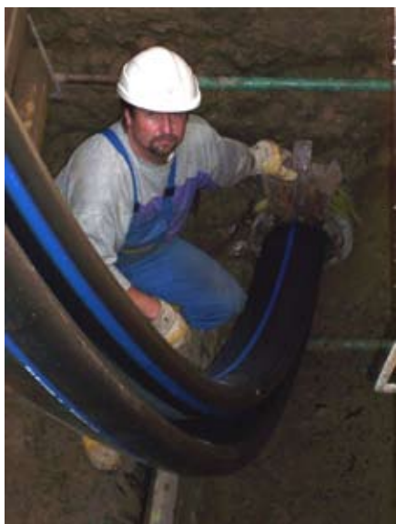
Pipeline renovation using close-fit technology. Photo: Roland Rohrhofer
